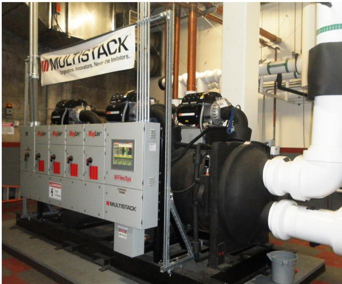
*“Multistack’s chiller has the air conditioning industry’s best unloading capability without the need for condenser water temperature relief...that’s amazing – a nominal 450-ton machine running in a stable condition at 40 tons. Technologically, that’s really a big deal. It’s a big deal economically, too. It is saving Universal a lot of electricity.”*
