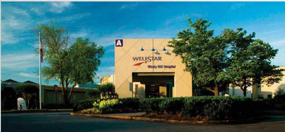
A part of WellStar Health Systems, Windy Hill Hospital opened in 1973.
