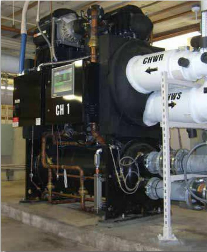
Moore Hall is equipped with two 160-ton Multistack chillers with the MagLev™ bearing system for high efficiency, high reliability and low maintenance.
