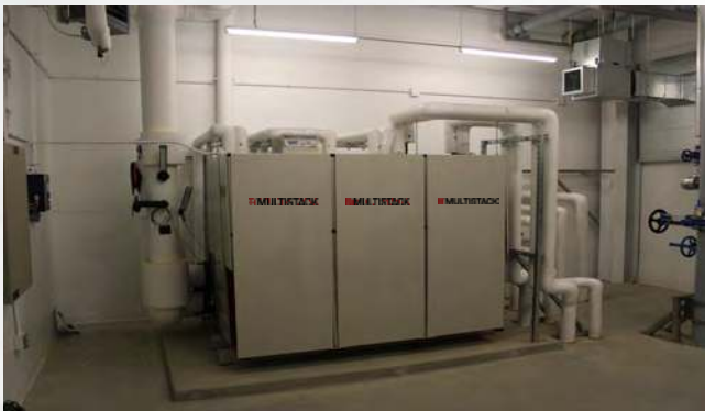
Three Multistack chiller modules, above, provide 140 tons of cooling capacity for The Spencer Brewery, right.
