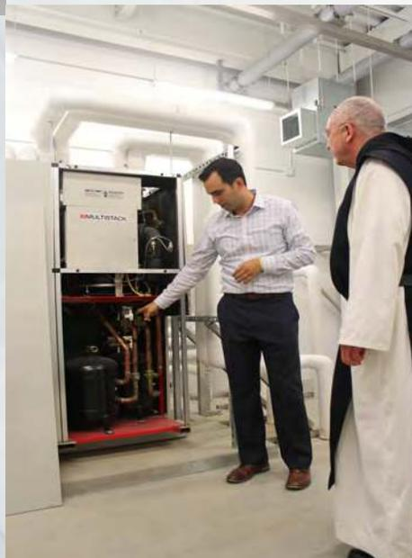
the modules and compressors needed to meet the load. And if a compressor should fail, the chiller has built-in redundancy.
