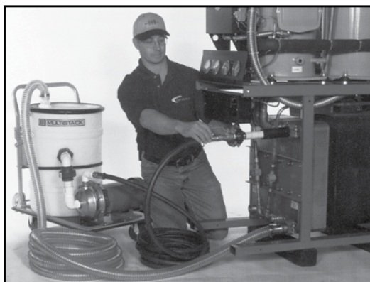
Figure 3, Inserting FlushGun into heat exchanger.
