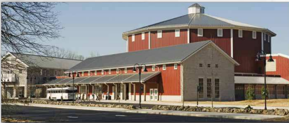
The Gettysburg National Military Park Visitors Center and Museum receives more than 1 million visitors each year. In 2010 it was awarded USGBC LEED Gold certification due to its energy-efficient geothermal HVAC system and other sustainable building design features.
