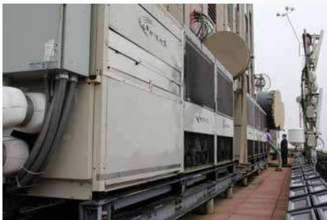
*Six 30-ton modules provide 180 tons of reliable, redundant cooling capacity for areas of the 80<sup>th</sup> and 86<sup>th</sup> floors at the Empire State Building.*
