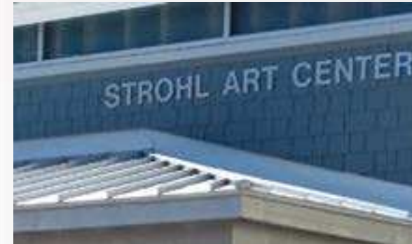
The Strohl Visual Arts Center and Fletcher Music Hall at Chautauqua Institution are both equipped with quiet, efficient Multistack air-cooled chillers. Photo courtesy of Chautauqua Institution.
