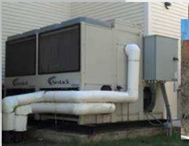
Above Left: A Multistack air-cooled packaged chiller serving the Strohl Art Center at Chautauqua Institution.
