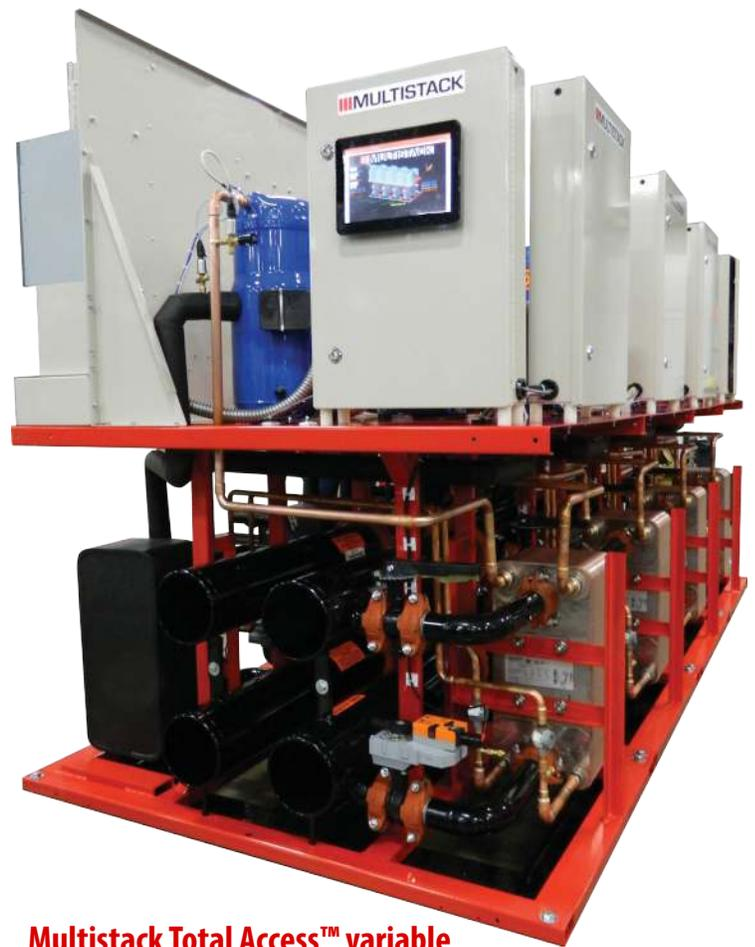
**Multistack Total Access™ variable speed chiller array with optional touchscreen display.**
