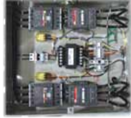
Multistack modules have an integrated digital controller, modulating source valve for head pressure control, thermal dispersion flow switch and over-current protection in each unit.
