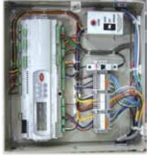
Multistack modules have an integrated digital controller, modulating source valve for head pressure control, thermal dispersion flow switch and over-current protection in each unit.
