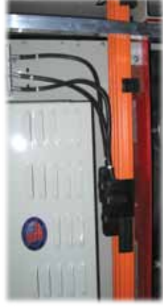
Single point electrical contact through a bus bar system standard
