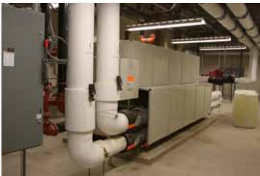
Water-cooled chiller installation.
