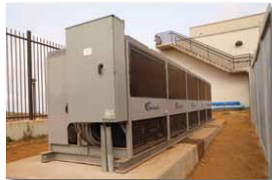
Air-cooled chiller installation.
